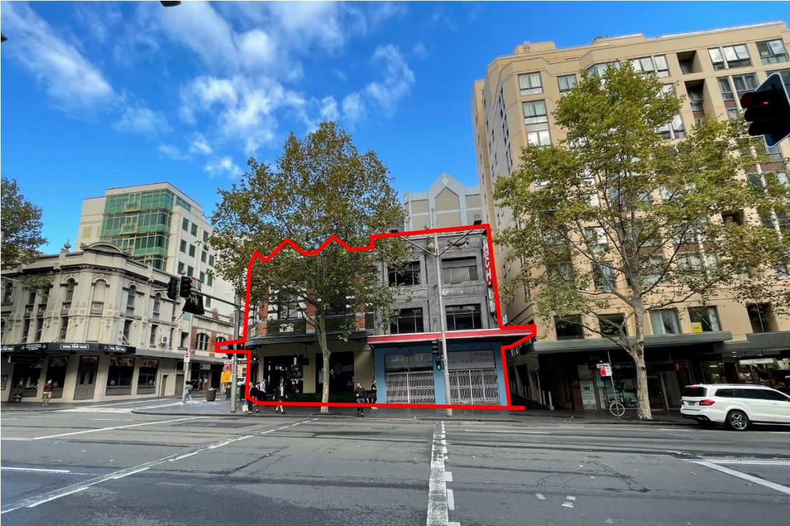
Figure 5. Looking west towards the 757-763 George Street sites, shown in red
